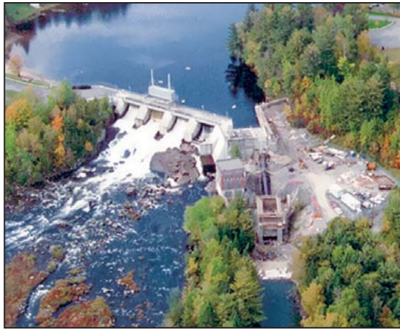
Figure 6: Small Hydro System.
