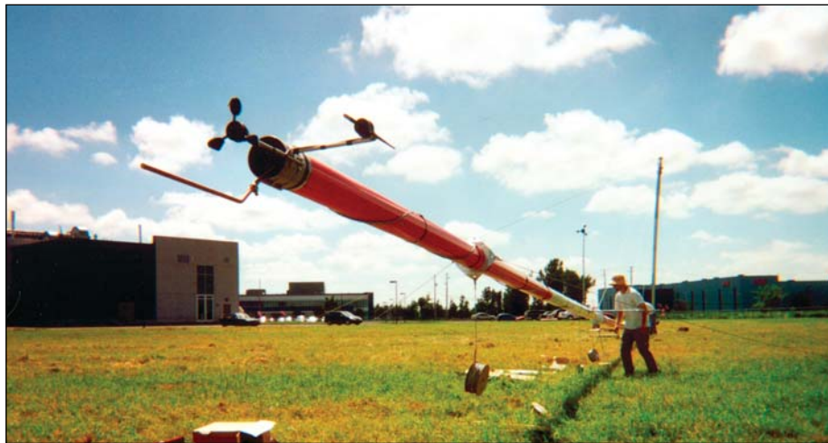
Figure 7: Installation of a 40 m Meteorological Mast.
