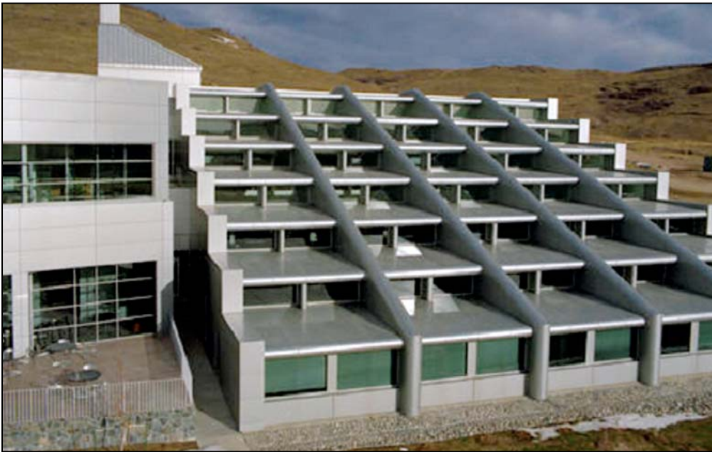
Figure 3: Passive Solar Design in a Commercial Building Application (NREL) in the United States.
