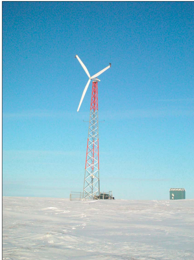
Figure 5: 50 kW Isolated-Grid Wind Turbine in the Arctic.
