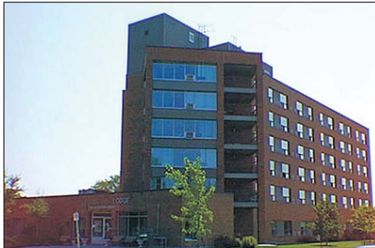
Figure 8: An Institutional Building Heated with Biomass.
