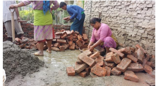
Recycling of bricks in mud mortar
