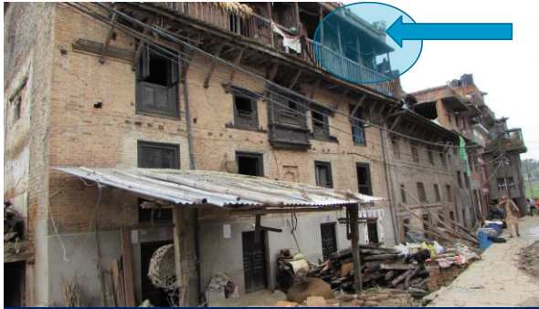
Addition of floors ( with RCC roofing in many cases)
