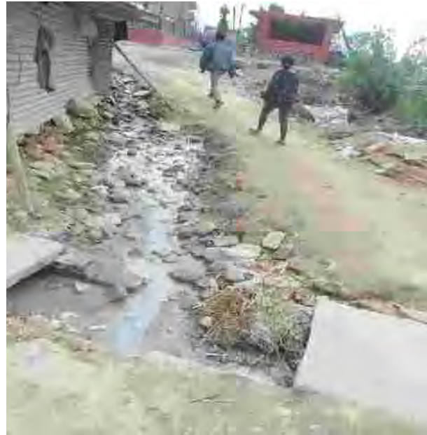
Fig2. Lack of maintenance of drainage system
