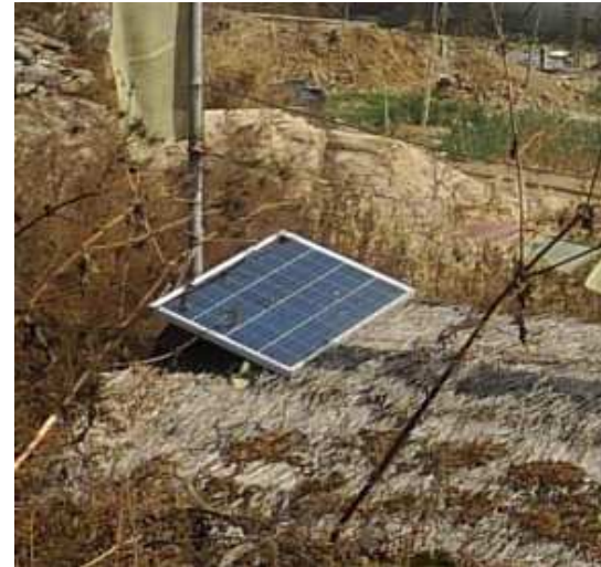
Solar PV panel small scale operation. Stand alone units.
