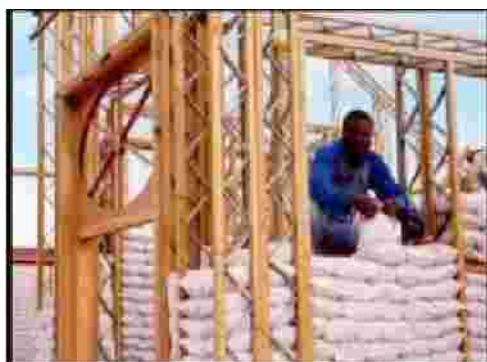
Figure 2: Eco-beam & sandbag construction, SA
