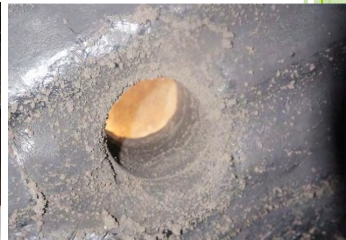
Fig: Hole in CGI Sheet functioning chimney
